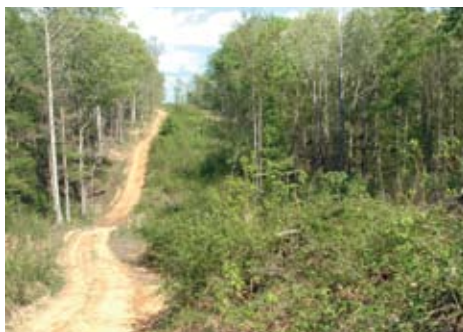
Fig. 12.2 This road has been daylighted on one side to produce additional browse for deer and nesting habitat for wild turkeys. The road itself has been graveled because it is traveled frequently.
